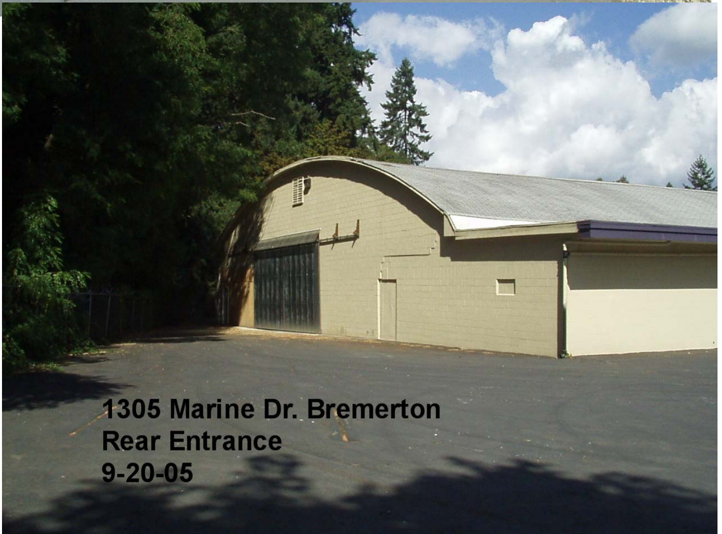
1305 Marine Dr. Bremerton Loading dock, office entrance 9-20-05
